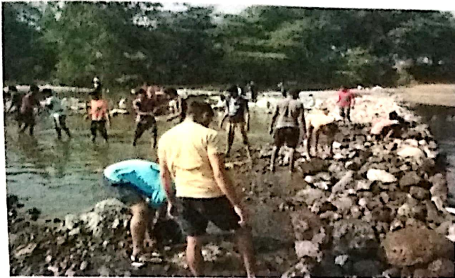
Construction of Bandhara at Bhima River
